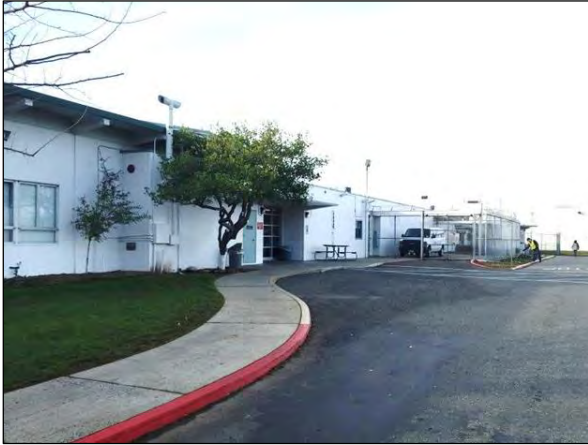
Butte County Jail Public Entrance and Adjacent Intake/Release Vehicle Sallyport
