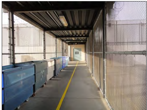
Exterior Circulation / Security Corridor between Main Jail and the West Facility
