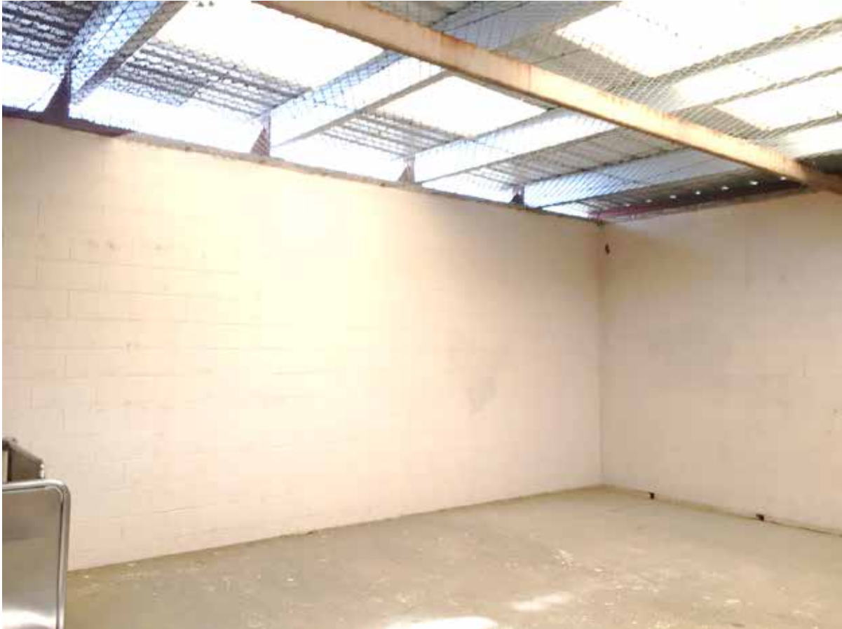
View of Quasi-Outdoor Recreation Yard
