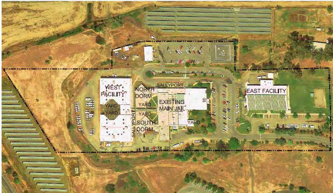
Aerial Photo of Butte County Jail
