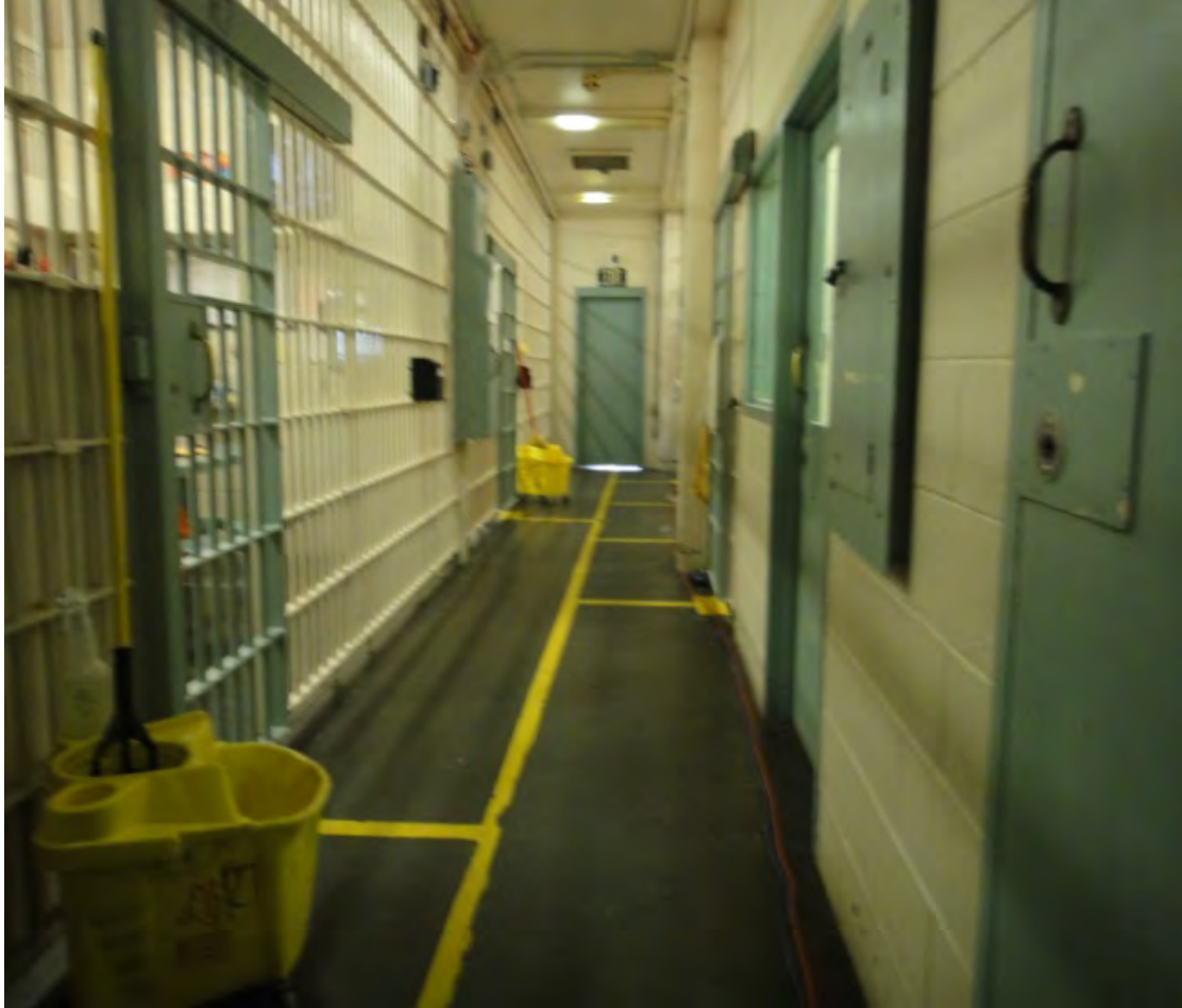
Main Jail Linear Female Housing With Barred-cell Fronts (Butte County is only one of a few jurisdictions still using this type of jail facility)
