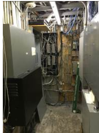
Electrical Room poses fire hazards
