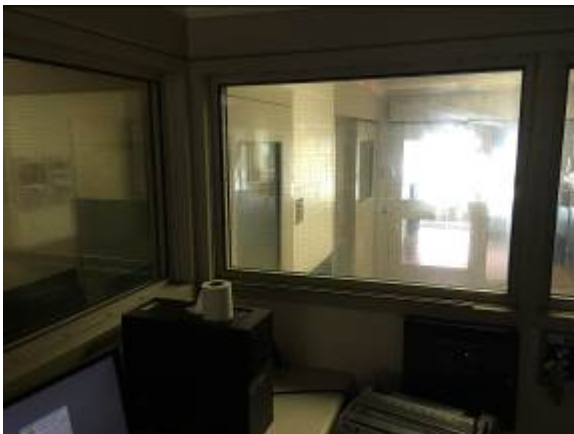
Glare on C1 Control Room windows
