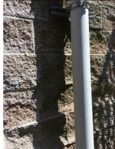
Roof drain no longer attached to wall as it has deteriorated the wall behind it.
