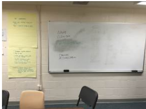
Whiteboard is old and needs to be replaced.
