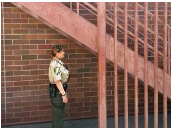
Head bump hazard under stairs
