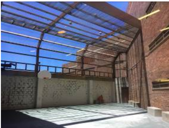
Balls are lost to roof covering.
