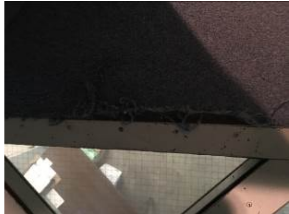
Carpet is approximately 15 years old. It is very frayed and presents tripping hazards in a dimly lit room.
