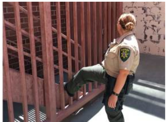
Inmates are able to climb the stairs in the Yard
