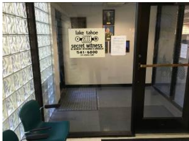
Glass block is poorly insulated
