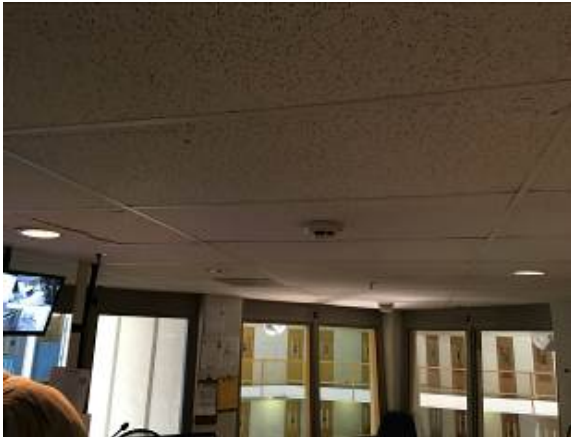
Lighting needs updated and replacing. Only 50% of the can lights in Modular Control currently work.
