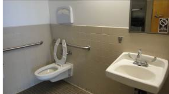
Unisex toilet is ADA accessible but not ADA compliant.
