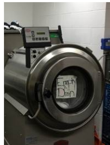
Posted reminder to empty drain to prevent overflow problems
