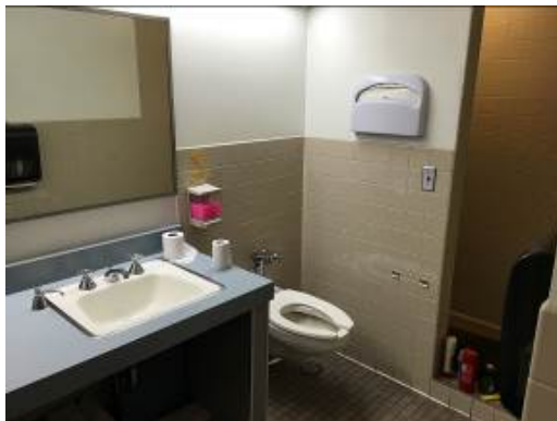
Staff Locker Room restrooms and showers are not ADA compliant
