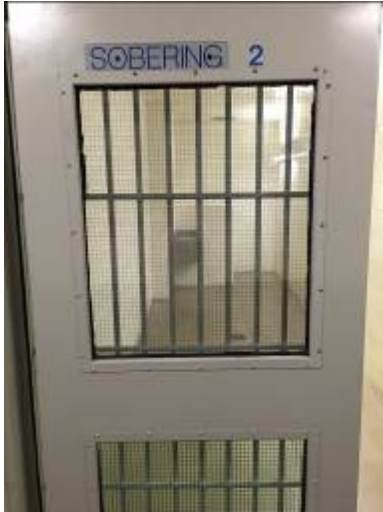
Sobering Cell bars present safety hazard
