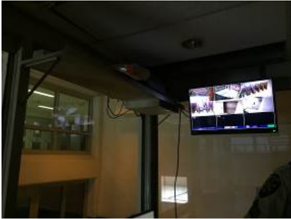
Additional monitors are needed to view cameras behind officer assigned to control
