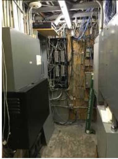
Exposed wiring in Electrical Room poses fire hazard
