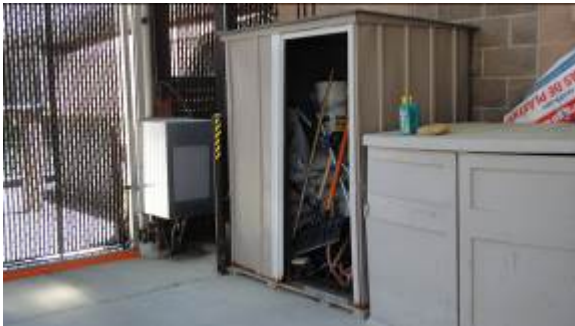
Tool shed doesn't close or lock.
