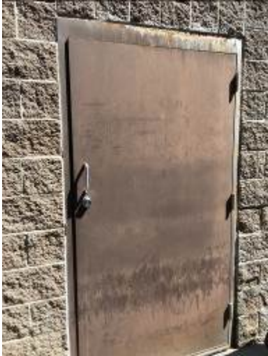
Unsecure door from Sallyport into Detention Aide office, allowing access to entire facility.
