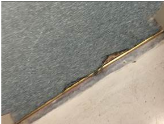
Carpet is frayed and needs to be replaced.
