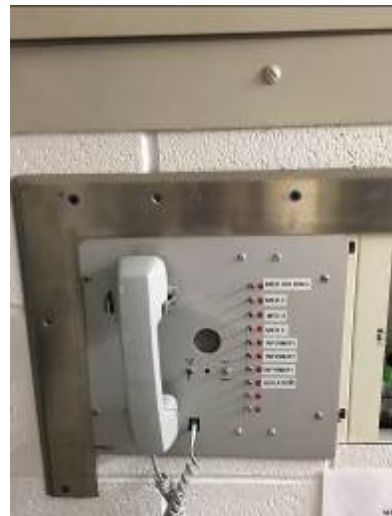
Intercom system that needs repair
