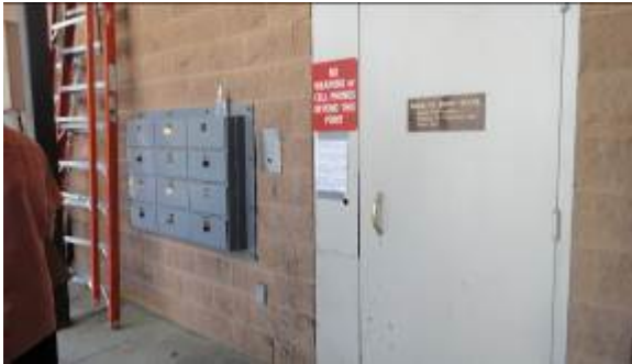
Gun lockers should be replaced with sliding doors as flaps are a major safety issue.
