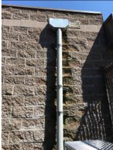
Roof drain freezes all the way down the wall in extreme cold conditions.
