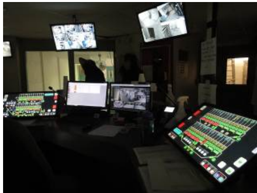
Television monitors for cameras are inadequate and larger monitors are needed.
