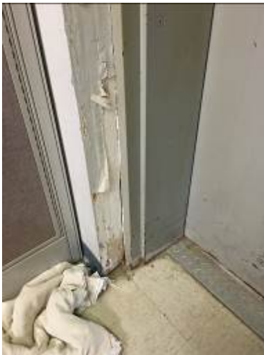
Water damaged door in Detention Aide office area
