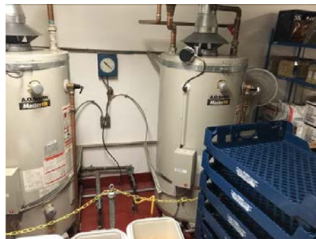
Water heaters in violation of Health Code
