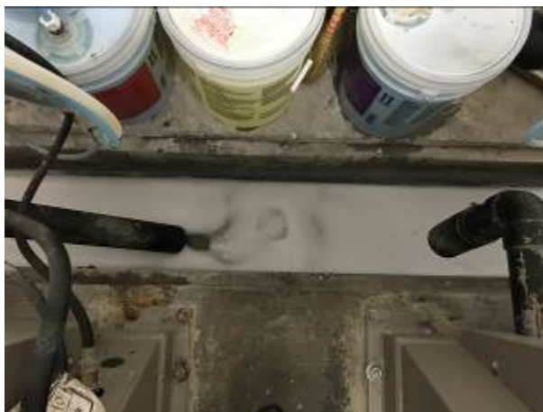
Laundry drain must be emptied 6 times per day
