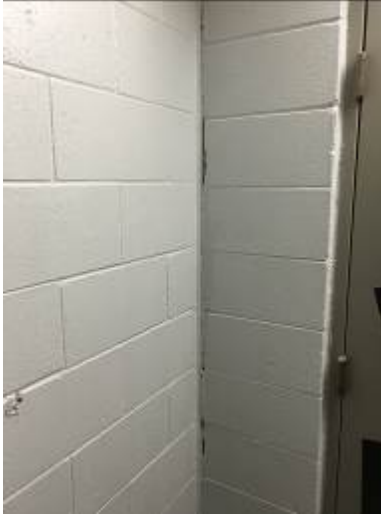
Cracks in walls hide contraband
