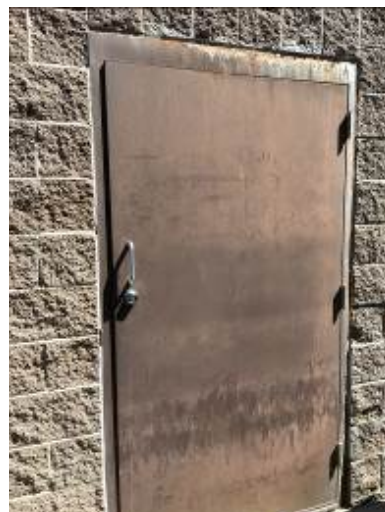
Sallyport door to Detention Aide office work space
