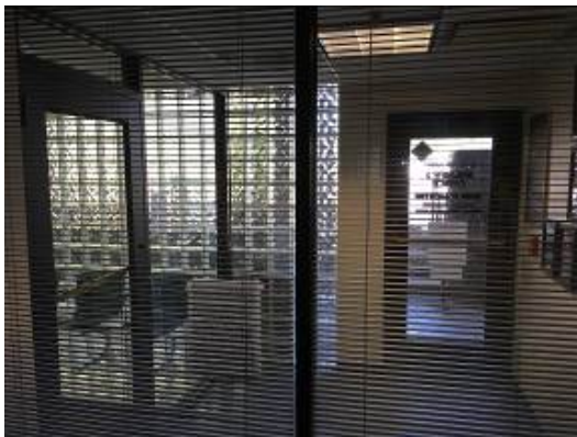
Receptionist is sitting behind drywall and regular glass that is not bullet proofed or secured.
