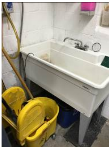
Sink area is small and difficult to maintain cleanliness
