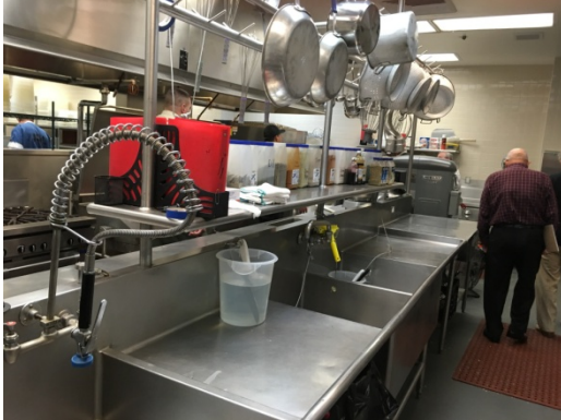
Placerville Jail Kitchen
