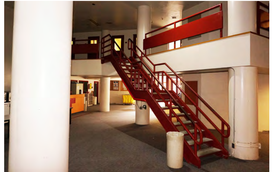
Figure 39: The typical housing unit is irregularly planned, with large structural concrete columns throughout, interfering with visual supervision.
