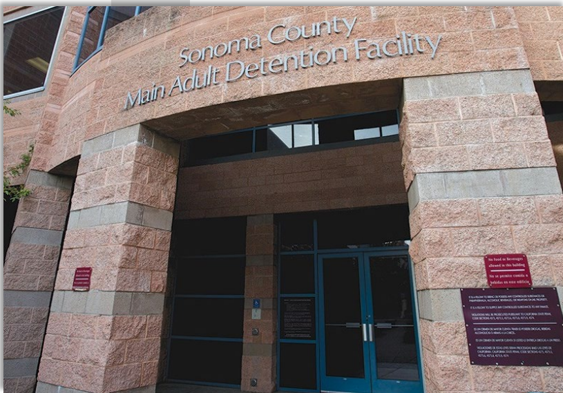
Main Adult Detention Facility
