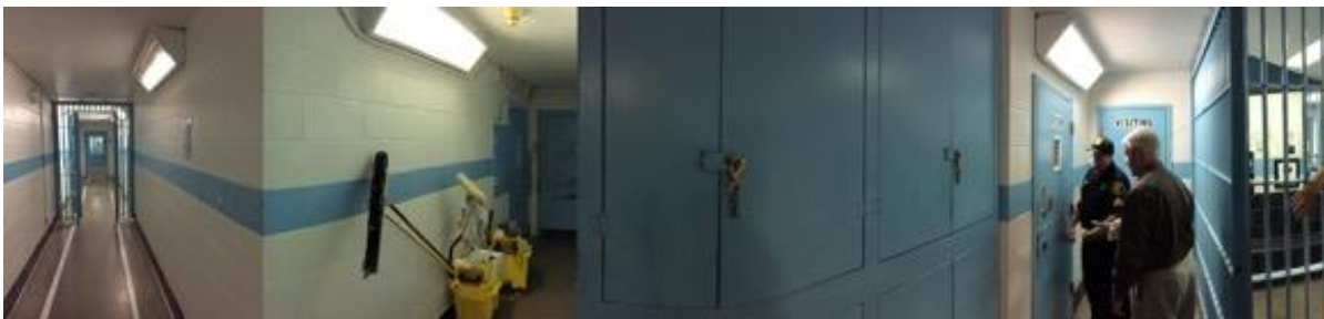
Primary Circulation from Intake to Support and Housing Spaces – Dangerous and Unsafe
